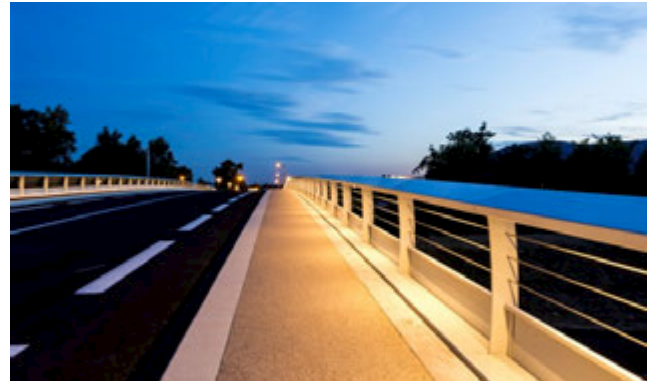
Outdoor – Example Bridge Lighting
