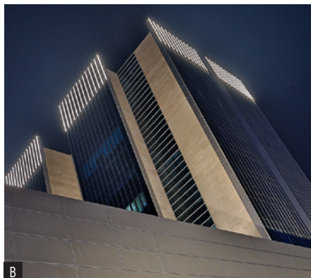
Eye-catching lines in high buildings
