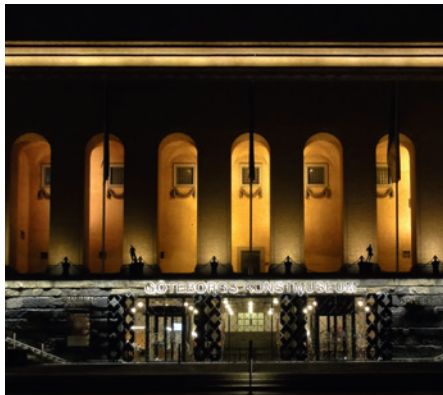
Efficiently highlighting wall structures
