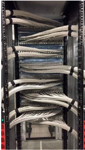
Proper rack cable management
