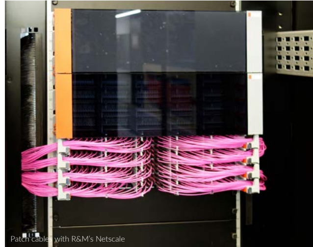
Patch cables with R&M's Netscale
