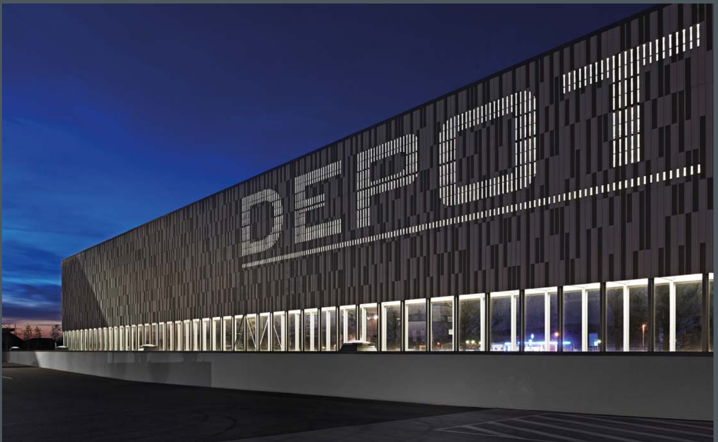
DEPOT noise protection wall, Niedernberg/Germany Lighting design: studiocandela, Herford
