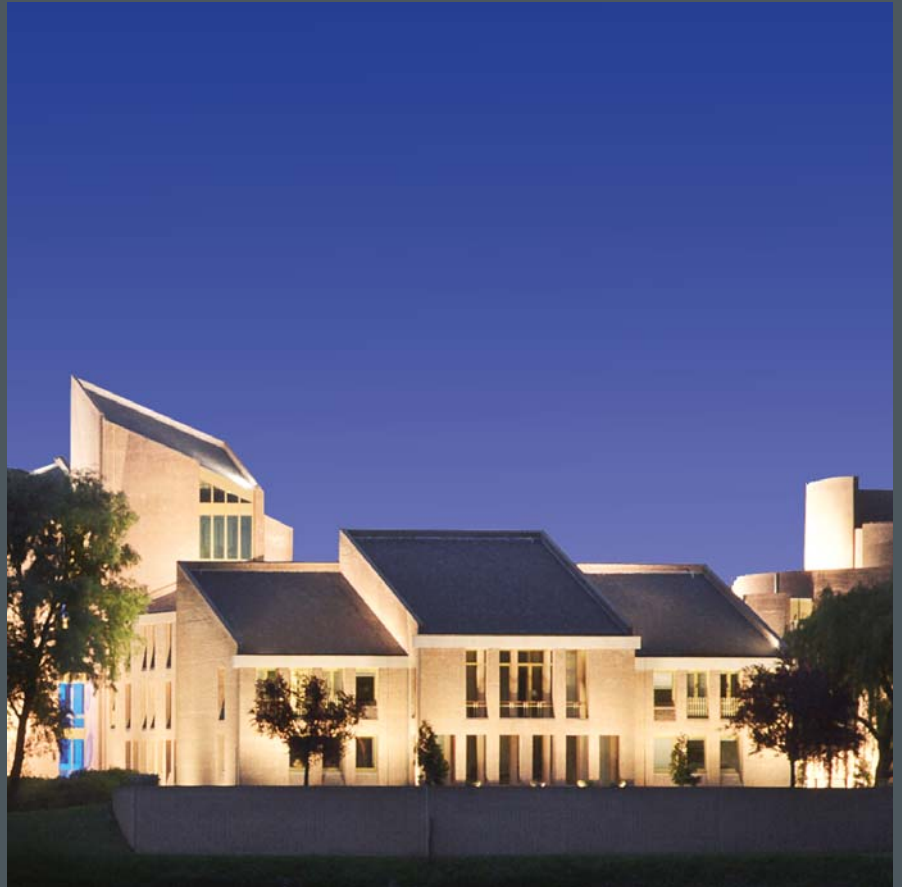
Province of Limburg's government building, Maastricht/Netherlands Lighting design: Studio DL, Hildesheim
