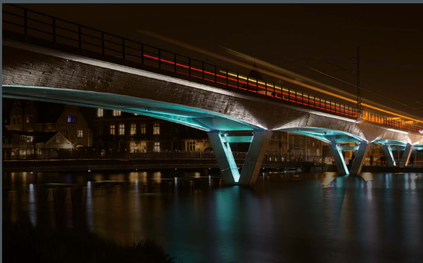
Railway Bridge, Eskilstuna/Sweden Lighting design: ÅF Lighting, Stockholm Photo by Sten Jansin
