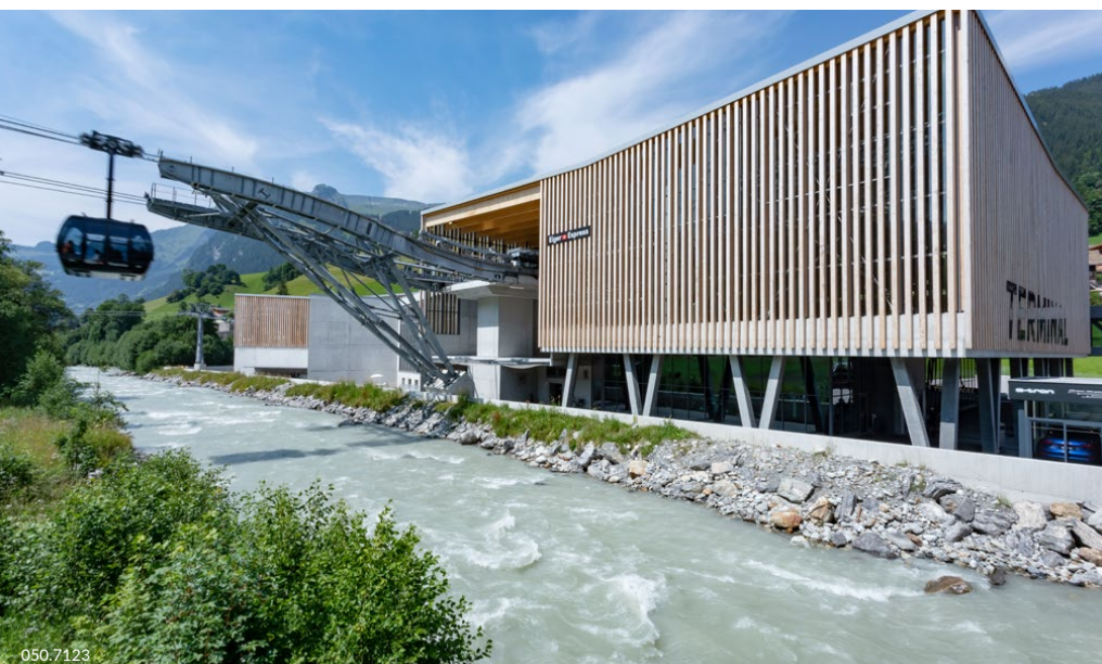
«Best Terminal in the Alps»: Wooden facade on the outside, a mobility center inside with digitized tourist operations on the inside – the new terminal in Grindelwald combines the Eiger Express, the Männlichen cableway, shopping, parking and access to public rail transport.
